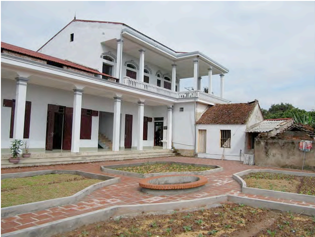
Photo showing completed construction at the HADC with improvements to grounds
